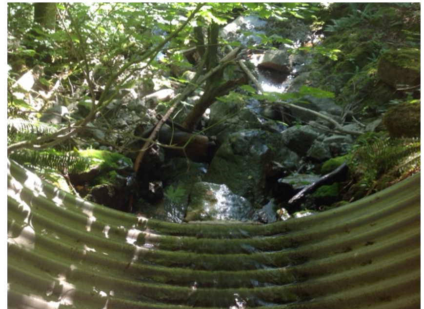
outlet from inside culvert
