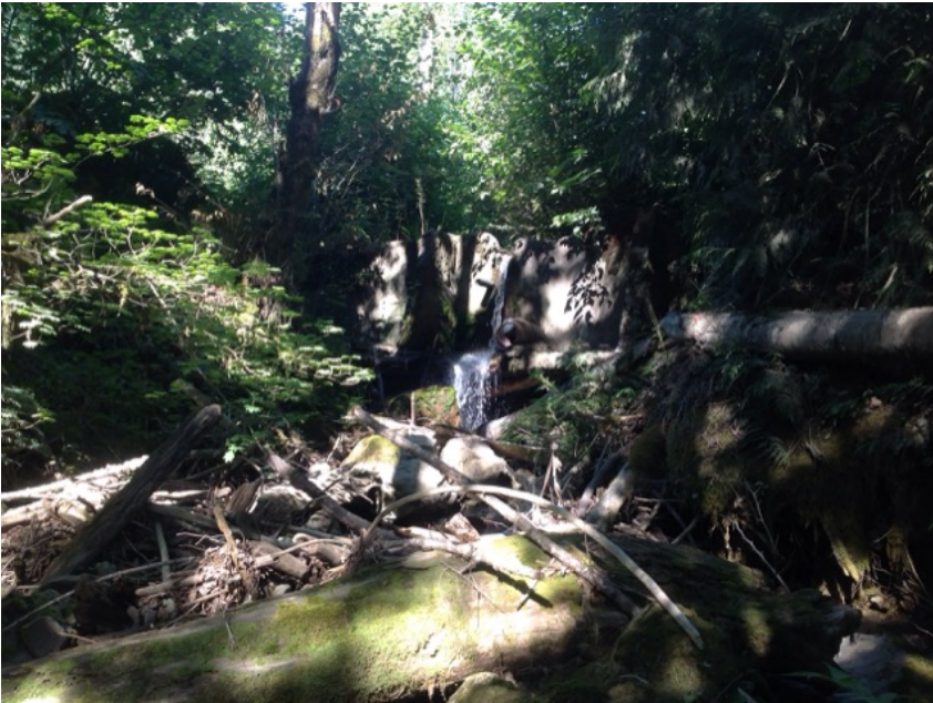
weir located 25 meters upstream from culvert
